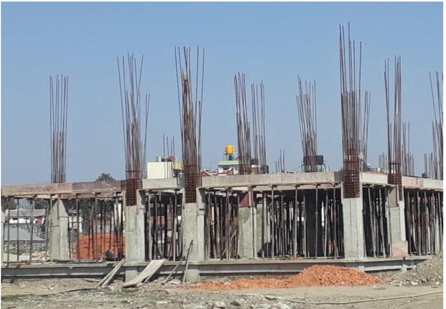
ATS Faculty Building under Construction
